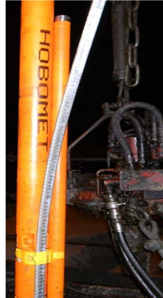
Bypass tube and pump
